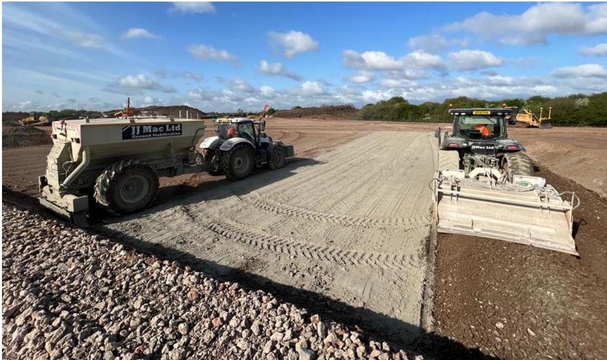
Water addition as necessary to ensure the Moisture Content Value MCV was within range at all times
