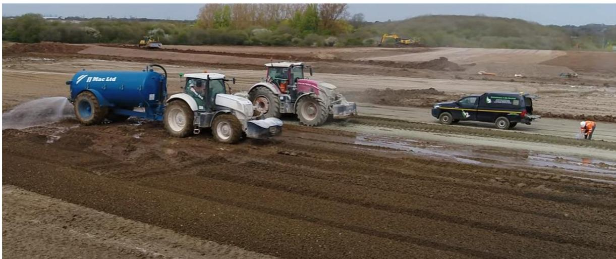
All works were tested during the construction process for MCV and CBR
